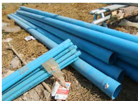
Water pipe connection
